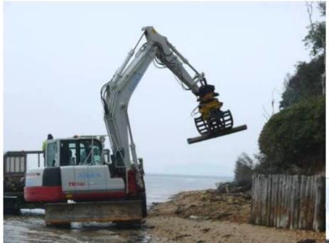
Removing some of the 2600 wooden piles & reprofiling the back scarp
